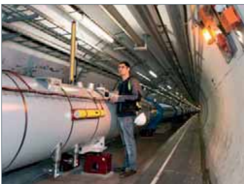
Nedo products in use at CERN
