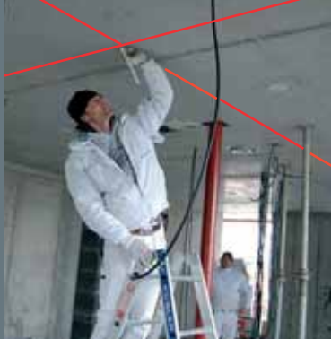
Simple transposition of plumb points and lines onto the ceiling.
